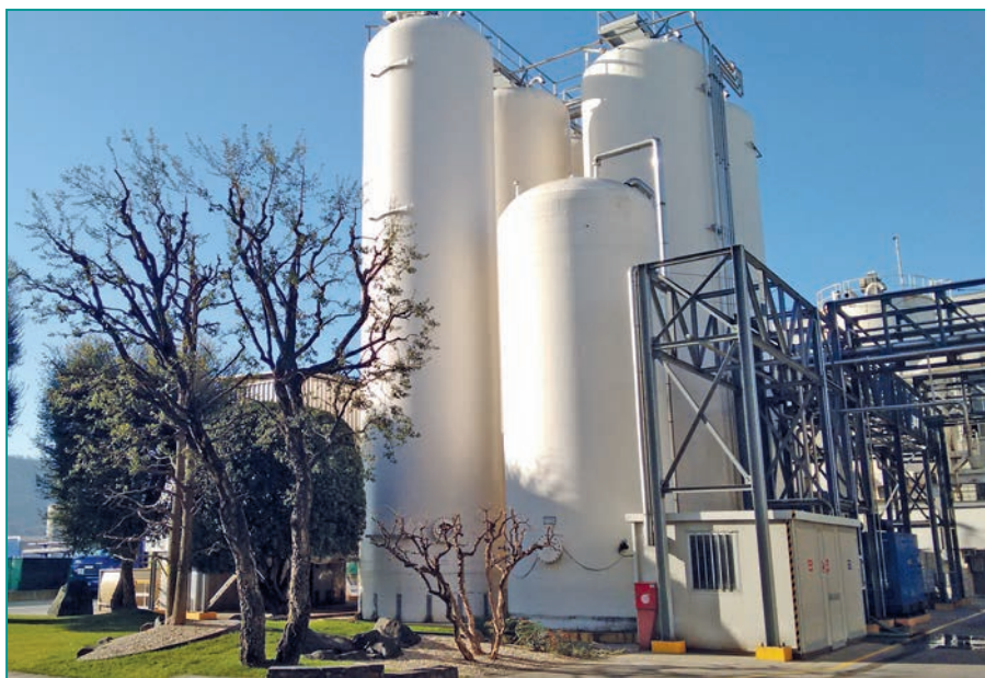
A SICIT production plant close to the tanning cluster at Arzignano-Chiampo in Italy, Credit: SICIT
