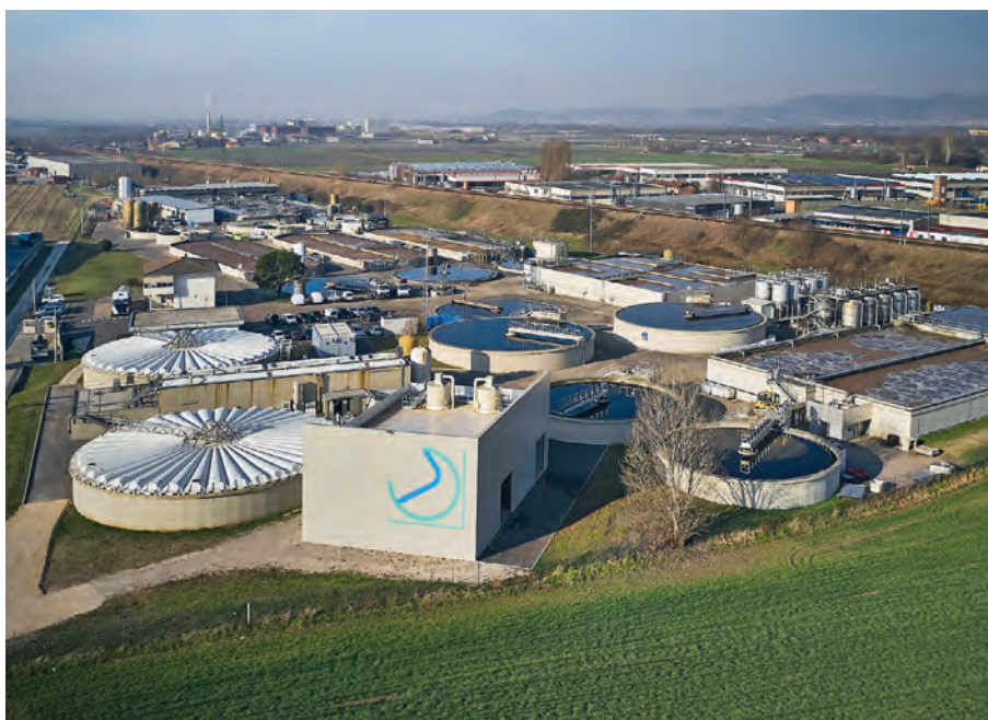
Wastewater treatment at Chiampo in Veneto. Water consumption in Italian tanneries has fallen by 13% in the last 20 years.
