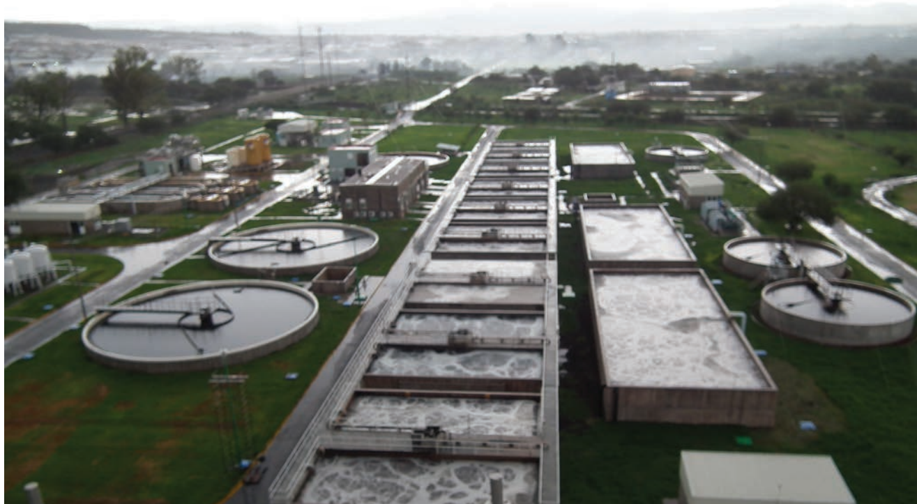
A water treatment plant in Guanajuato. Other footwear-making states, such as Jalisco, face a more challenging water environment.
