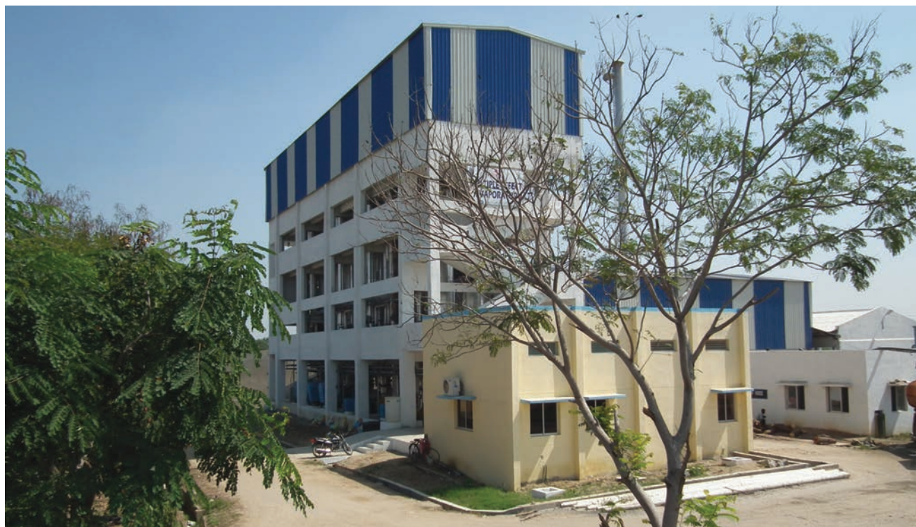
CETP plant, Ranipet. ALL IMAGES: WTP
