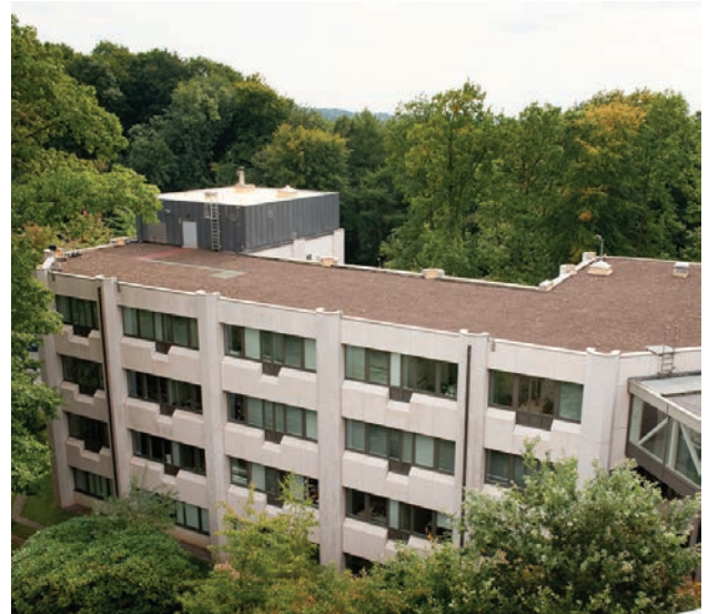
Huntsman's research and development centre for footwear at Everberg in Belgium. CREDIT: HUNTSMAN
