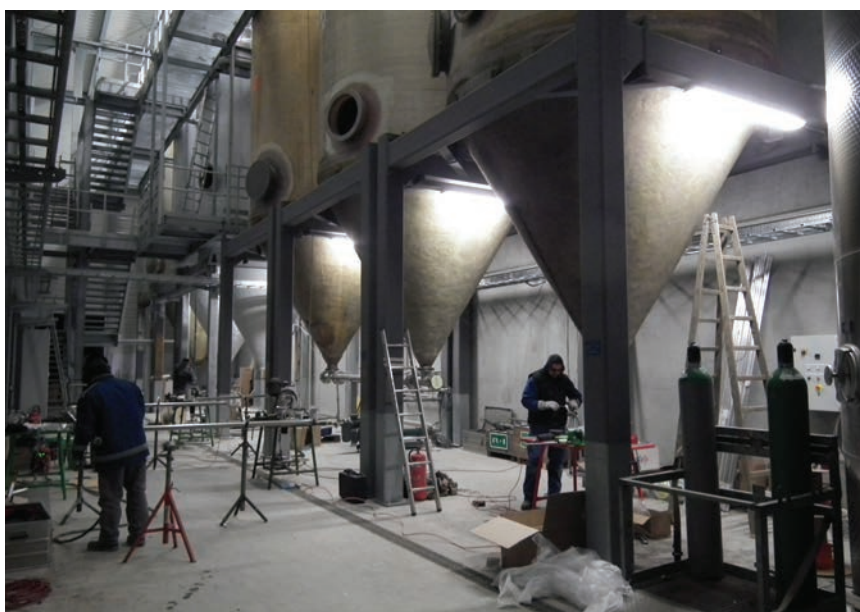
Recycling, reduce and reuse are very much part of modern tanning. These settling vessels being installed in a tannery in Austria are designed for the recovery of proteins, following the acid precipitation of unhairing/liming wastewaters and washings after sulphide removal.
